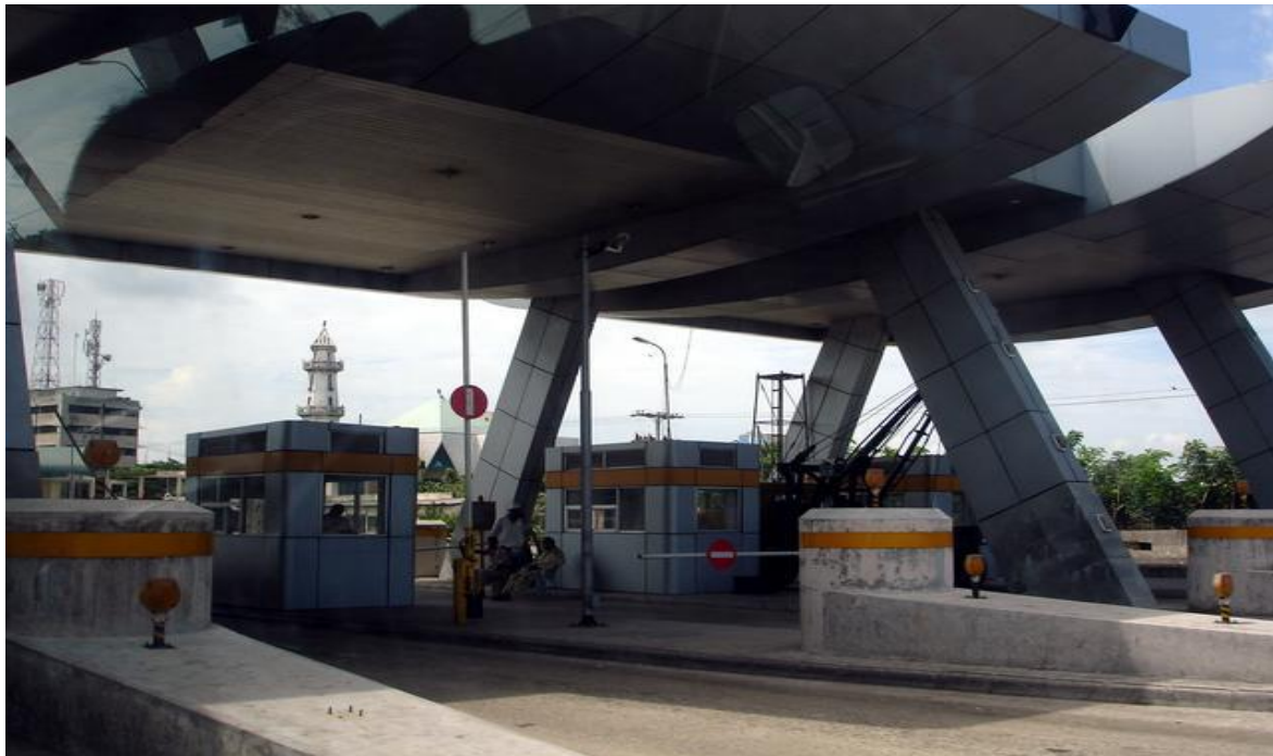
2.1. Figure: Proposed area, Meghna Bridge Toll booth
