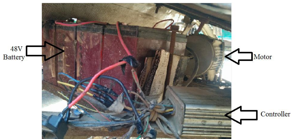
Figure 8.3: Electric vehicle equipments
