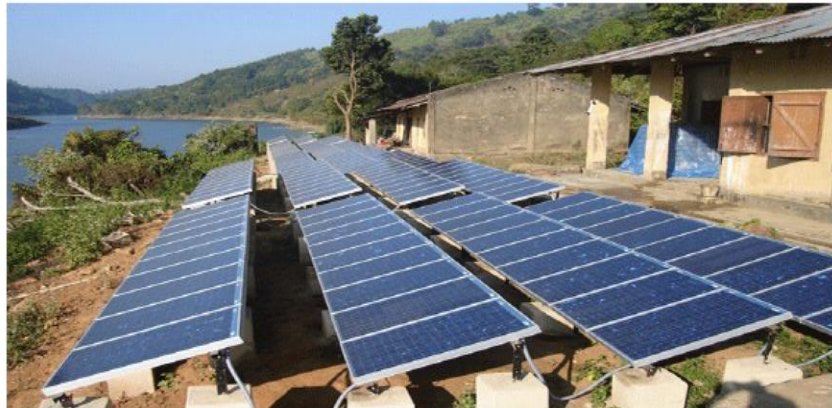
Figure 2.7: Solar Arrays of 10 kWp Centralized AC Market Electrification System at BarkalUpazila under Rangamati District
