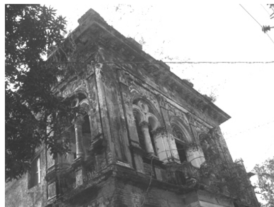
Figure 9: Buildings like this should be revitalized or preserved, Source: Iftekhar Ahmed (2003)
