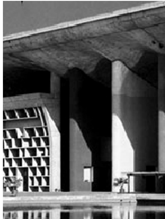
Figure 22 Walls, High Court
