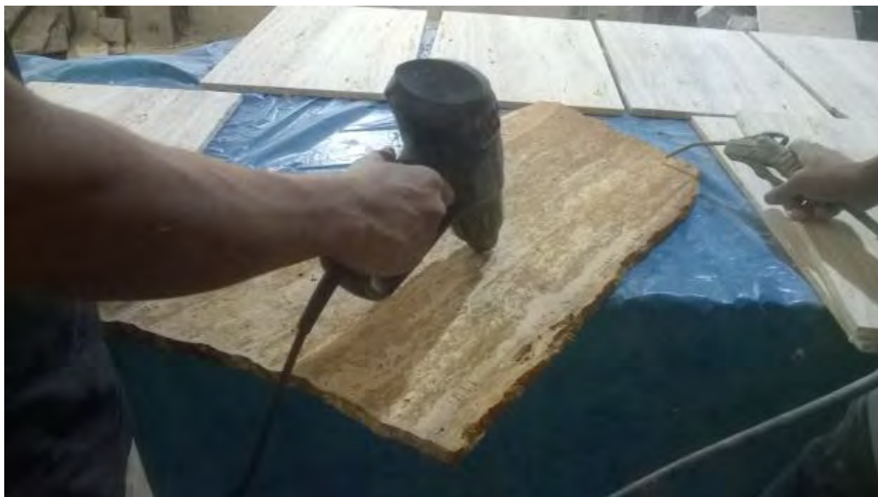
Filling the gapes with glue of travertine
