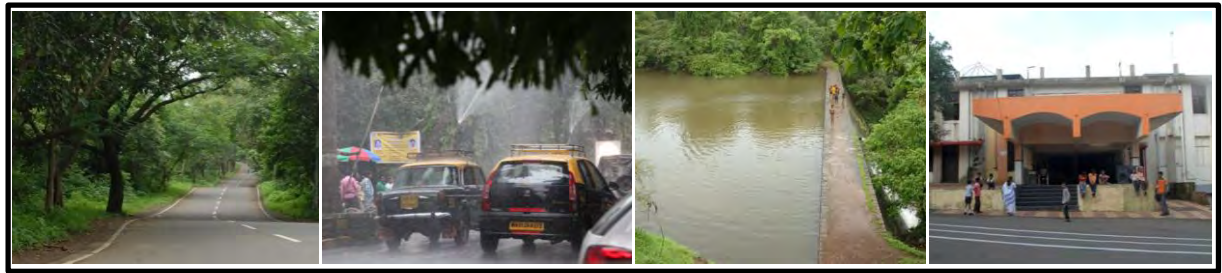
Fig.4.2.3: Built conditions inside the Mumbai Film City
