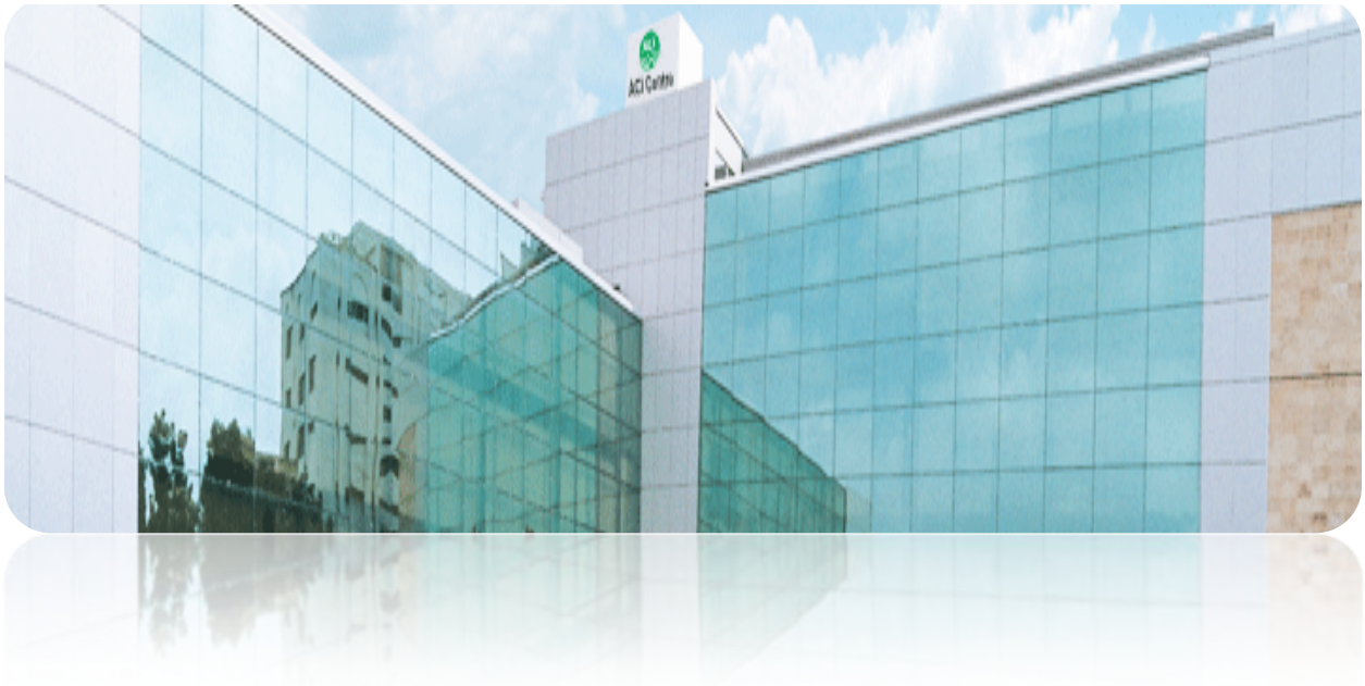
ACI Center (Head Office)
