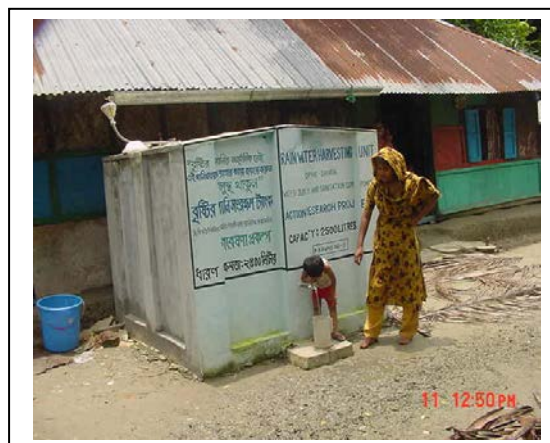
Figure: 2.4-Rain Water Harvesting
