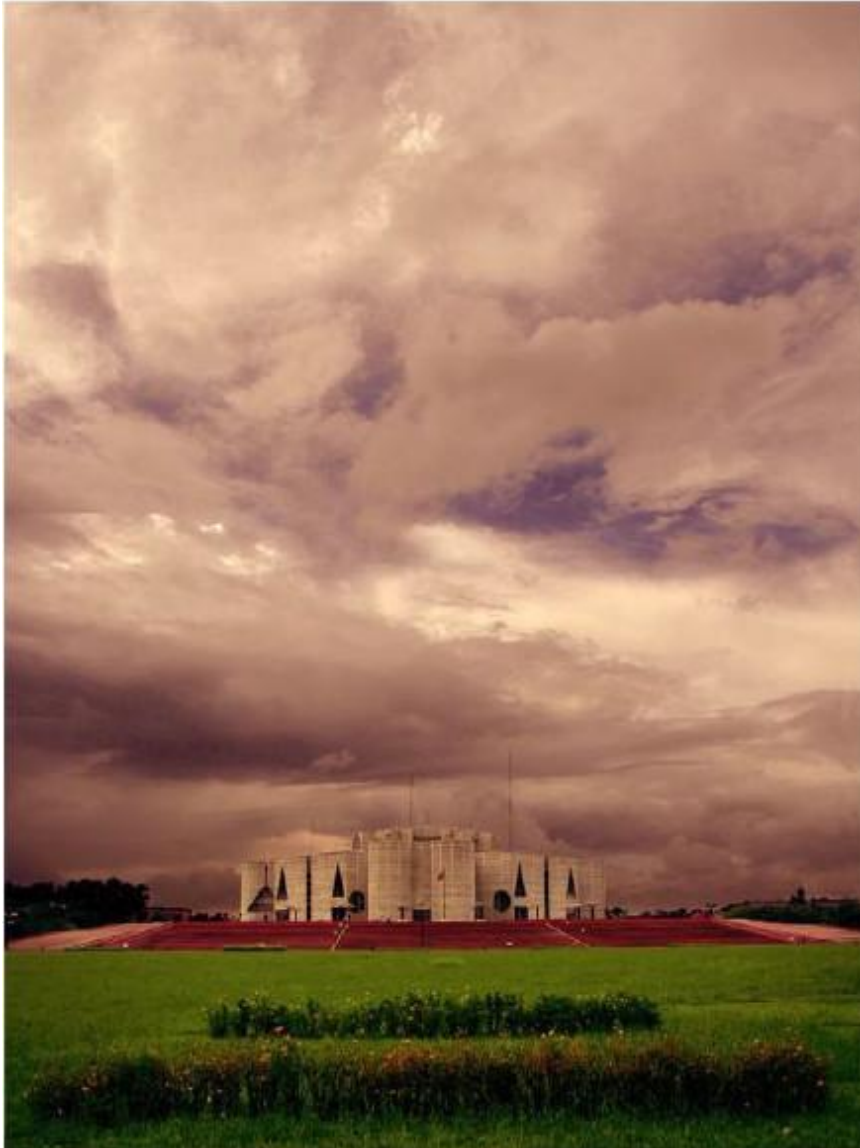
Fig: 5.7- The National Assembly Building at the heart of lush of green.
