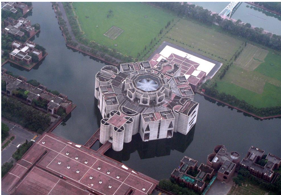
Fig: 5.8- The National Assembly Building surrounded by water.
