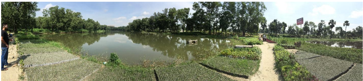
Fig 2.3- Site images showing the current conditions of the site.
