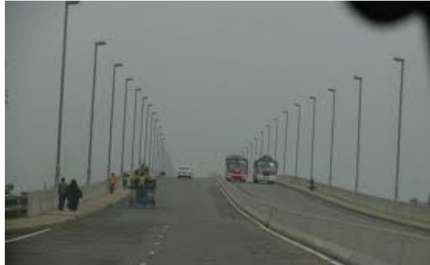
Picture: Vhairab Bridge
