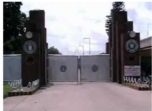
GTCL Compressor Station, Char Chartala, Asuganj
