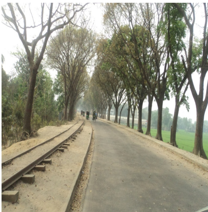
Dhaka-Sylhet Highway to Fertilizer Industries Connecting Road in Char Chartala
