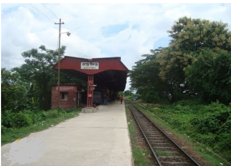
Asuganj Rail Station
