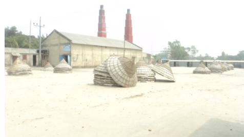
Picture: Boiler Based Rice Husking Mill
