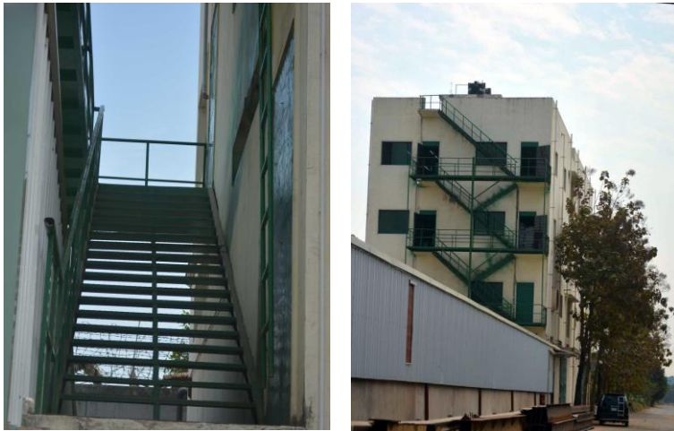
Figure 45 & 46: Fire escape stair of queen south factory.
