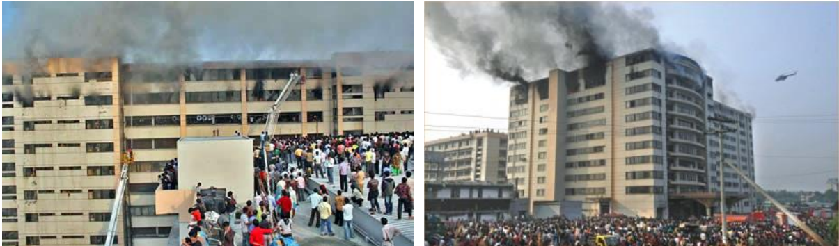
Figure 22: Fire hazard in Ha-Meem Factory.
