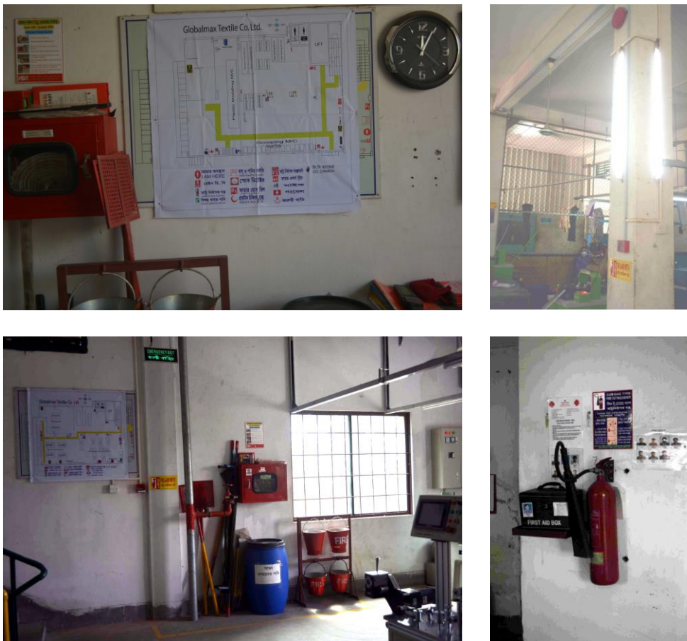
Figure 47 -50: Escape route layout & firefighting equipments.
