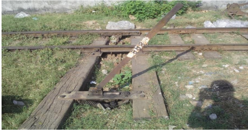
Fig 1.4: Manual Hand Lever based track switching system
