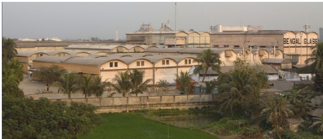
Fig 2.1.1: Factory Building, located east of Dhaka city, along the Shitalakya River
