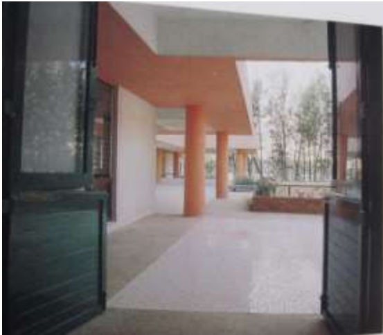
Fig 54 The upper level looking at the river
