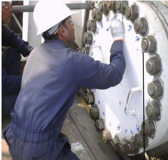
Here the technicians are performing Star/Cross pattern marking and hand tightening the bolts
