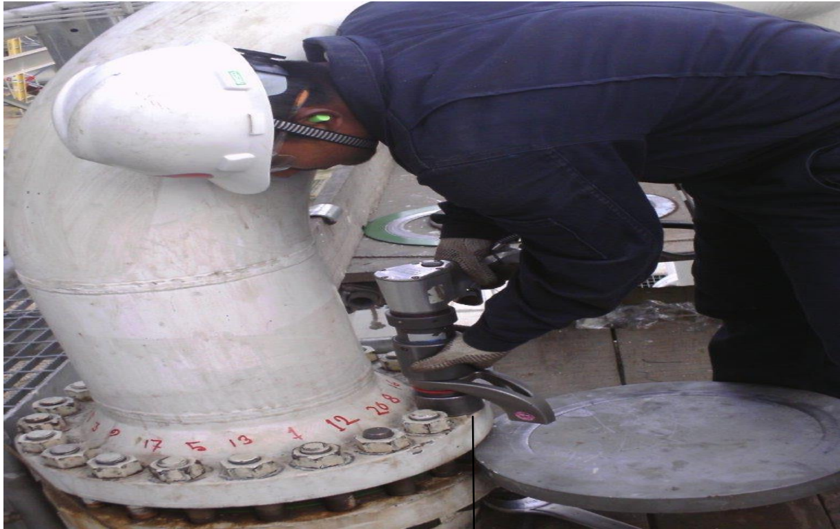
Here the technician is applying final torque using a torque gun
