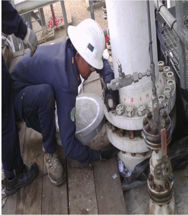
Here the technicians are swinging the spectacle for both isolation and de-isolation
