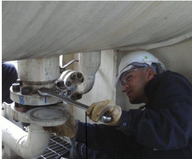
Here the technicians are performing Star/Cross pattern marking and hand tightening the bolts
