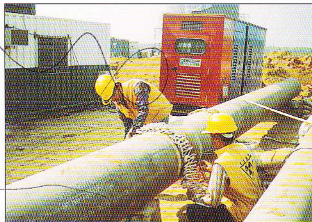
Installing induction heating coil for PWHT (Stress Relieving)
