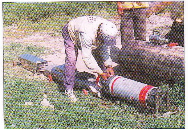
Assembling X-Ray crawler before put into work
