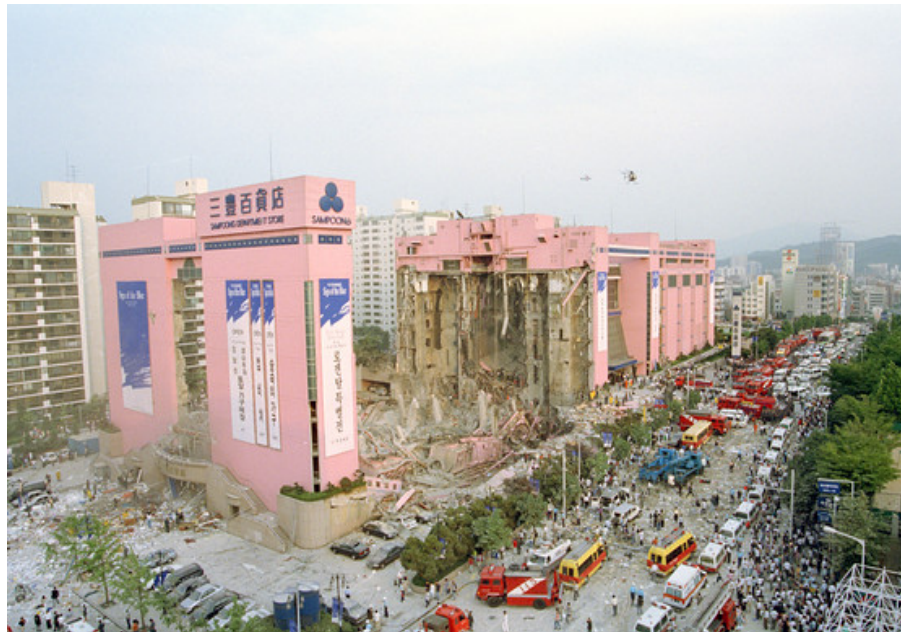
Figure 2.3: Collapse of Sampoong Department Store in June 29, 1995. (Source: http://blogs.wsj.com/korearealtime/2014/02/18/south-koreas-history-of-building-collapses/ )
