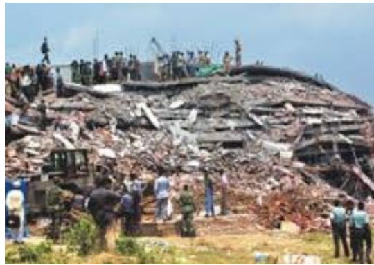
Figure 2.5: debris of Spectrum Sweater factory
