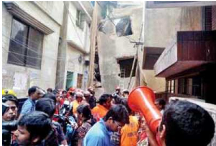
Figure 2.4: Shakhari Bazar building Collapse, 2004 at old Dhaka city (Source: http://www.thefinancialexpress-bd.com/old/index.php?ref=MjBfMTBfMDNfMTJfMV8yXzE0NTYyNg== )
