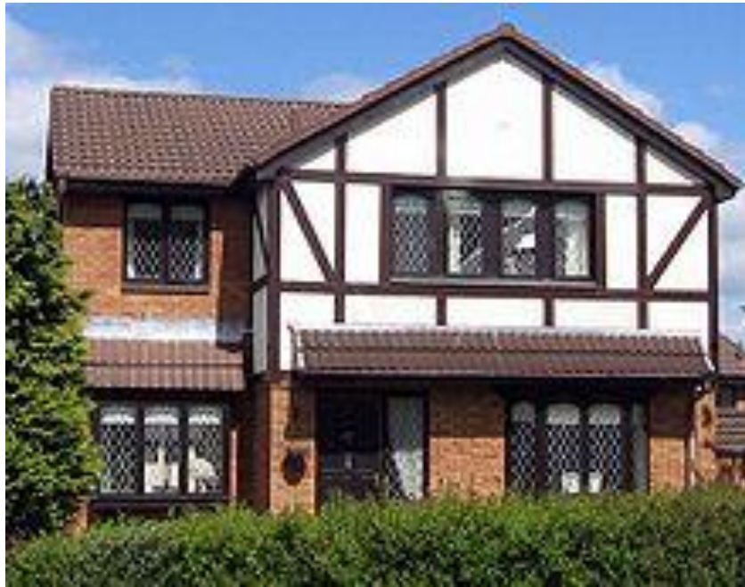
"A modern Tudorbethan" house with uPVC gutters and downspouts, fascia, decorative imitation "half-timbering", windows, and doors
