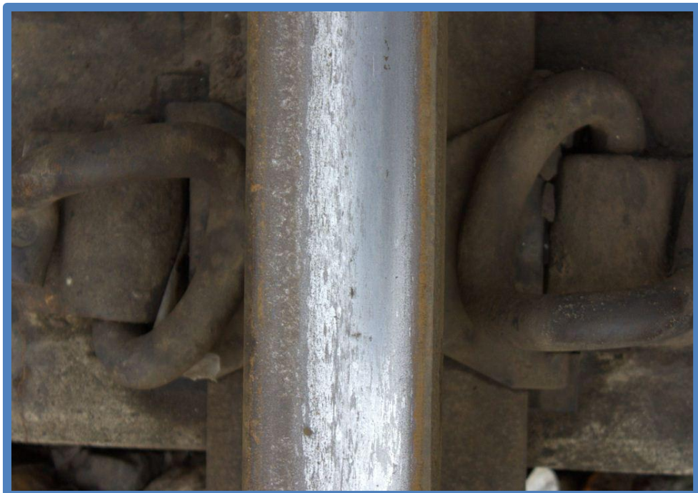
FIG: 1.2 Rail line without expansion joint gap
