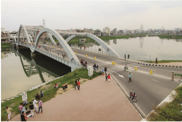
FIGURE 02 (a): Image towards a connecting bridge
