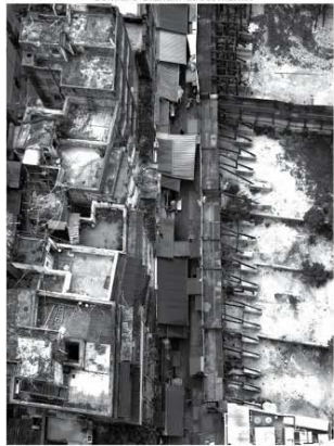
4. Graham Street, Central: current condition with open-air wet market, urban block on right demolished.
