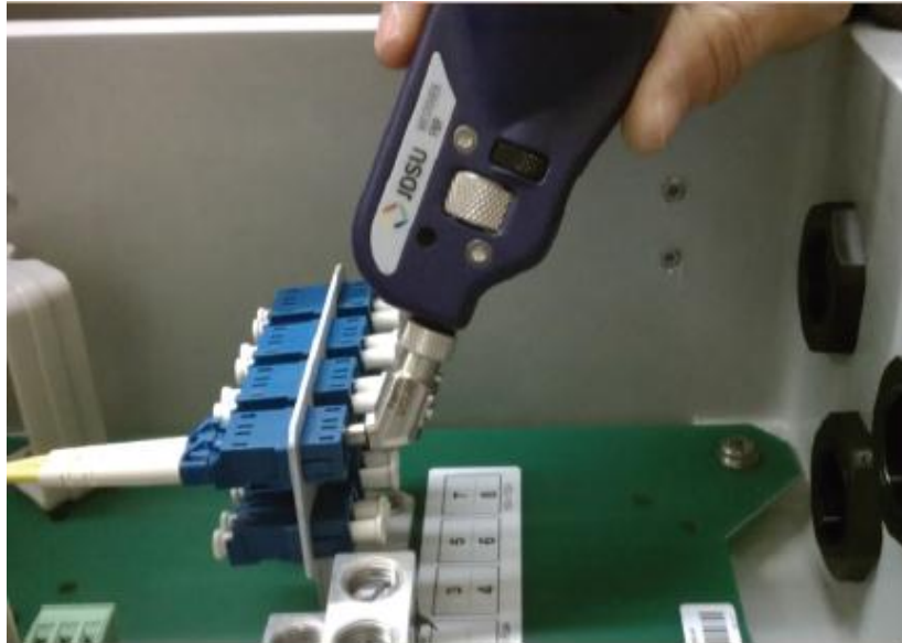
Figure 6.22: Connectors Inspected Before Installation [44]
