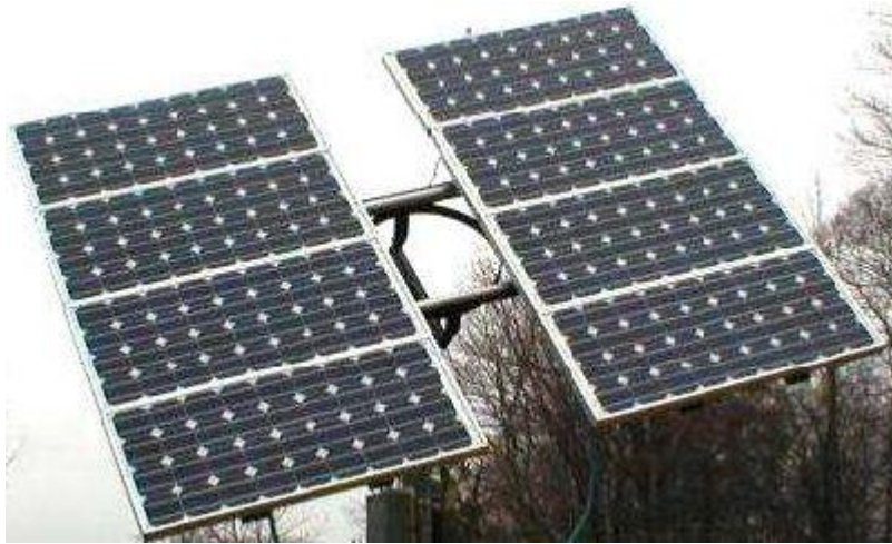
Figure: 14 Dual Axis Tracker
