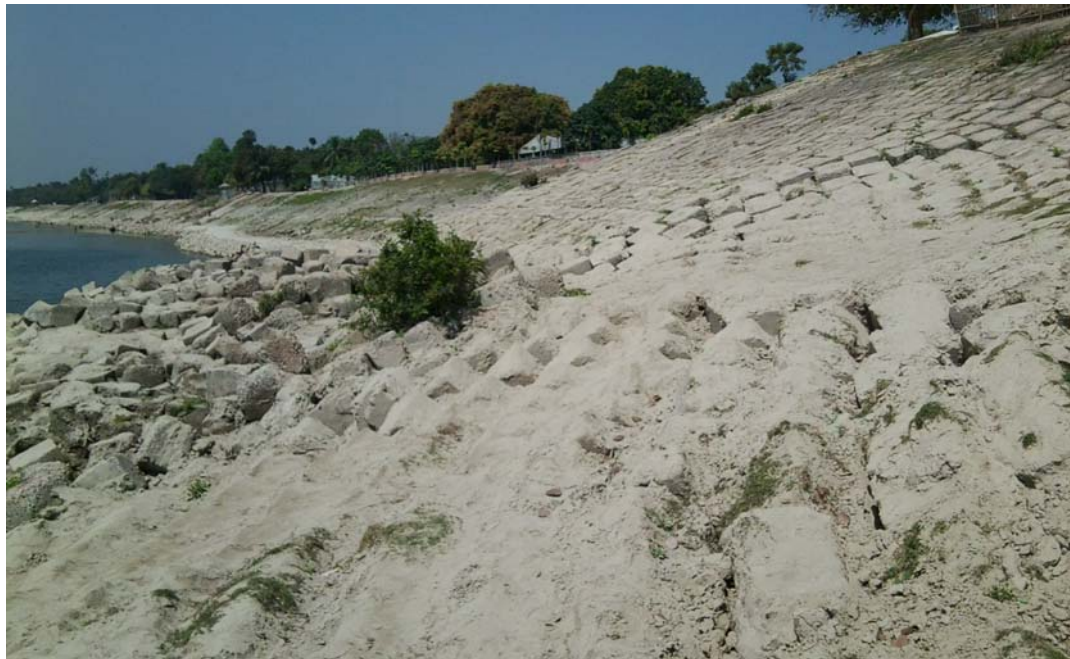
Figure 4.6 Revetments from Kundupara to Baruria
