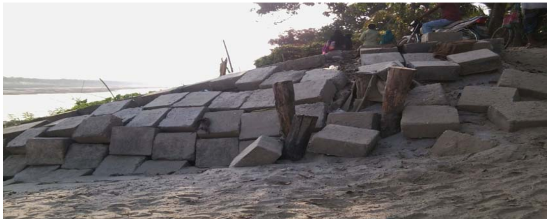
Figure 4.8 Revetment at Elongi
