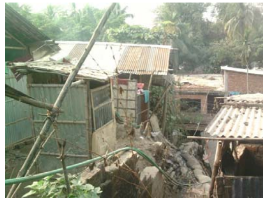
Fig: 4.17 Unsafe latrine Source: Author, 2013
