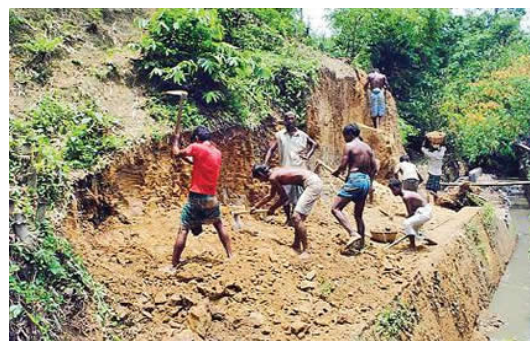
Fig: 2.3 Hill cutting for road expansion Source: Dainik Notunbarta, 10 June 2013
