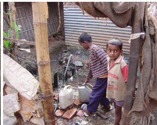
Fig: 4.11 Illegal stand pipe of water Source: URB.im
