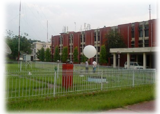
Figure1. 4: Weather Station analog sensors
