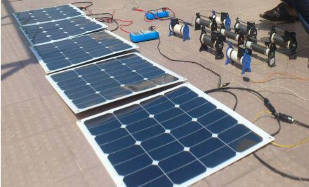
FIGURE 3.1: The 50 W semi flexible solar panels used for the project
