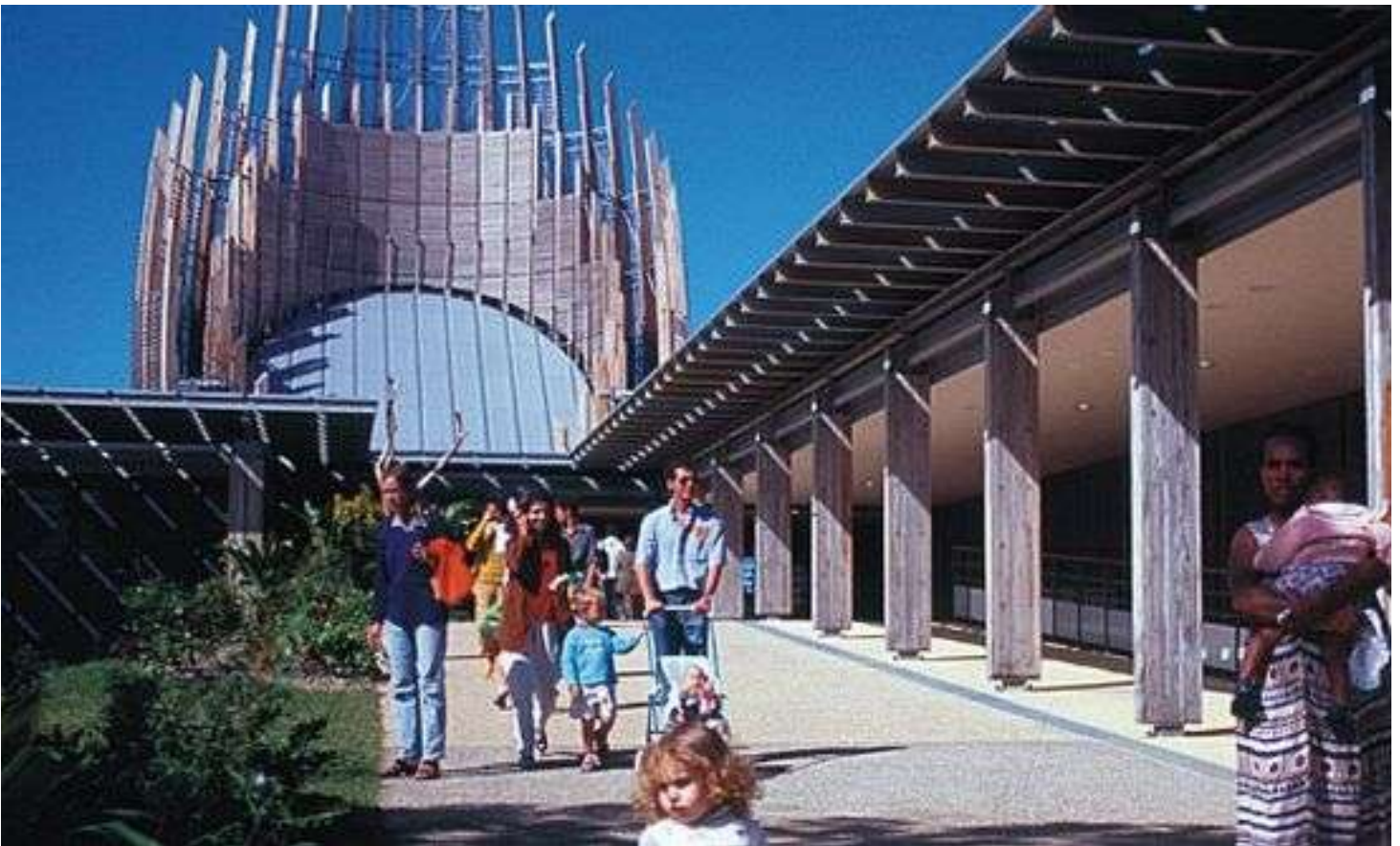
Figure 4.2.14: Covered walkway, view from courtyard
