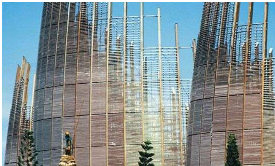
Figure 4.2.11(b): Exterior Facade
