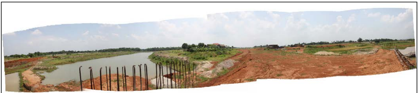
IMAGE 5: IMAGE OF THE EXISTING CONDITION OF THE SITE
