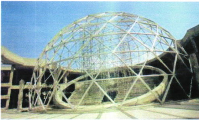
Figure 5:- Construction of Novo Theatre
