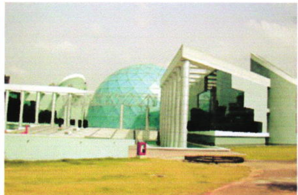
Figure 6:- View After Completion Of Work
