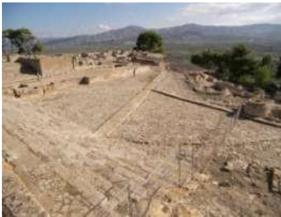
Figure 6: Rainwater Harvesting in Palace of Phaistos (Mays, 2012), an open yard to collect the runoff water is shown on the left, and a special cistern with a sandy filter is shown on the right.
