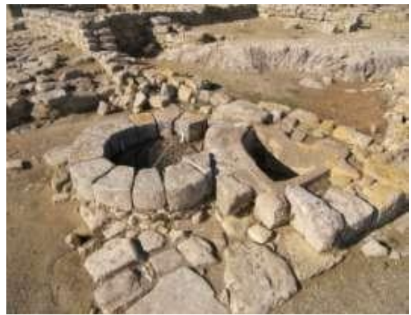
Figure 6: Rainwater Harvesting in Palace of Phaistos (Mays, 2012), an open yard to collect the runoff water is shown on the left, and a special cistern with a sandy filter is shown on the right.
