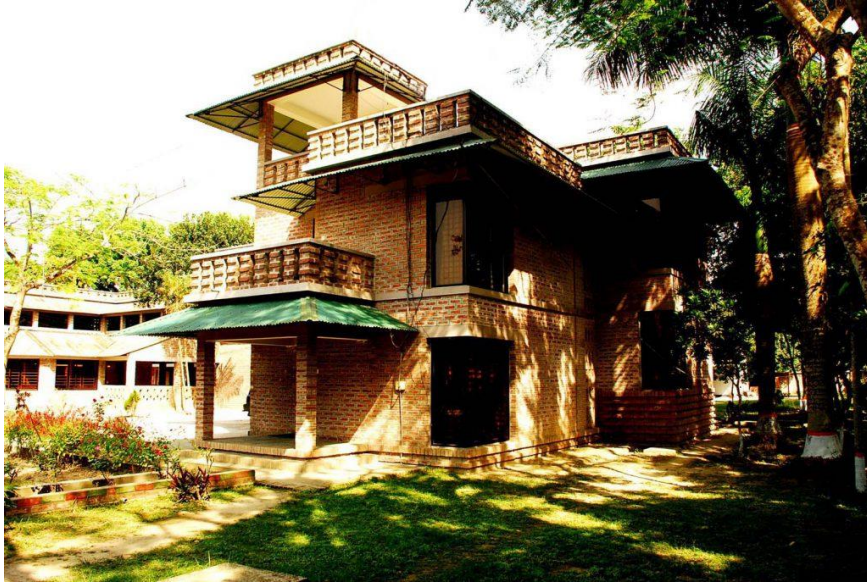
Figure 16: Cluster of accommodation facility
