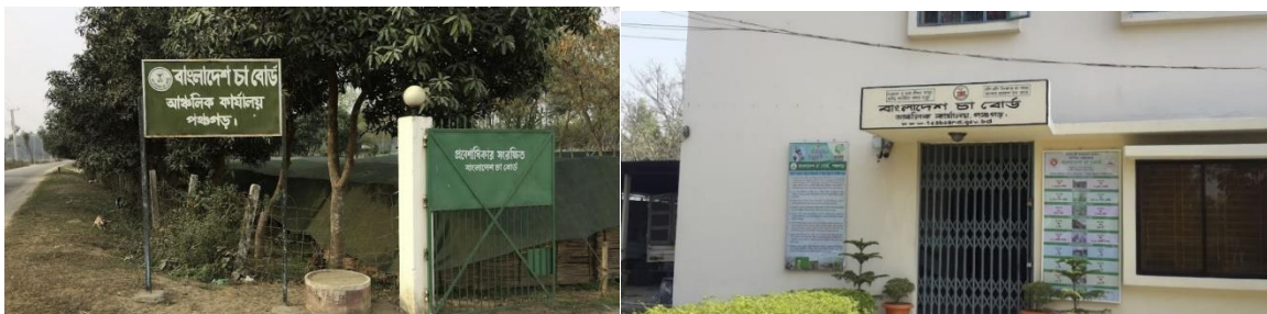
Fig 23: Existing buildings of the site | source: author
