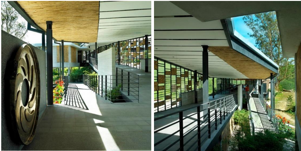
Fig 35: Roof materials, BOH visitor center | source: arch daily
