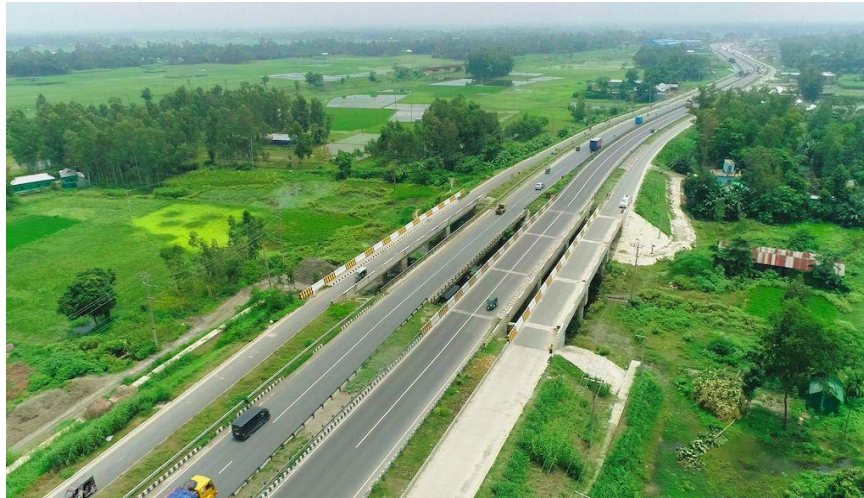
Fig 4: Dhaka -Tangail four lane highway with separated service lane under SASEC project
