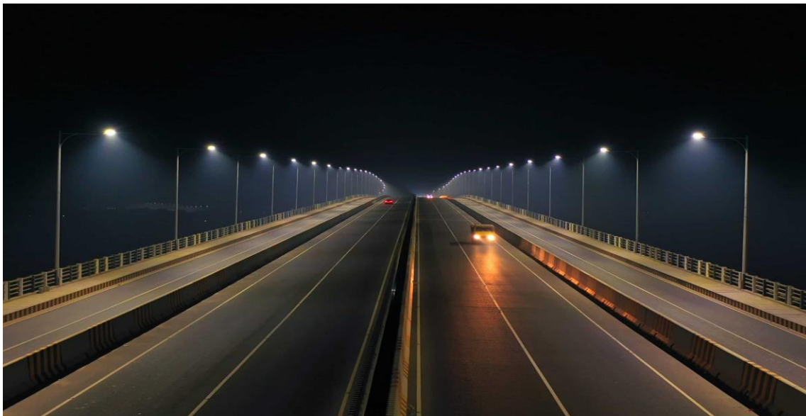
Fig 5: Dhaka mawa Expressway (Photo captured 2022)
