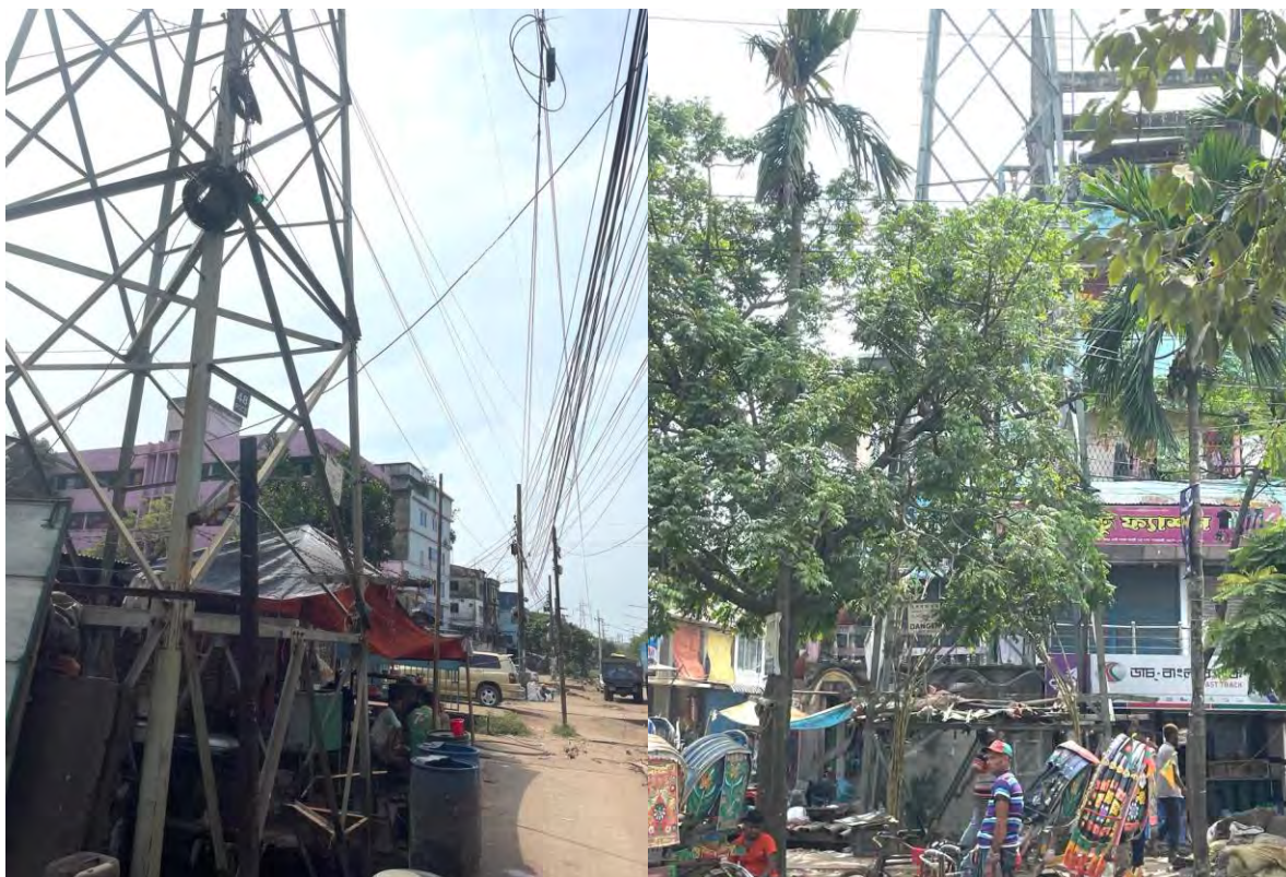
Figure 7: Habitats located dangerously close to cell towers in the city of Chittagong
