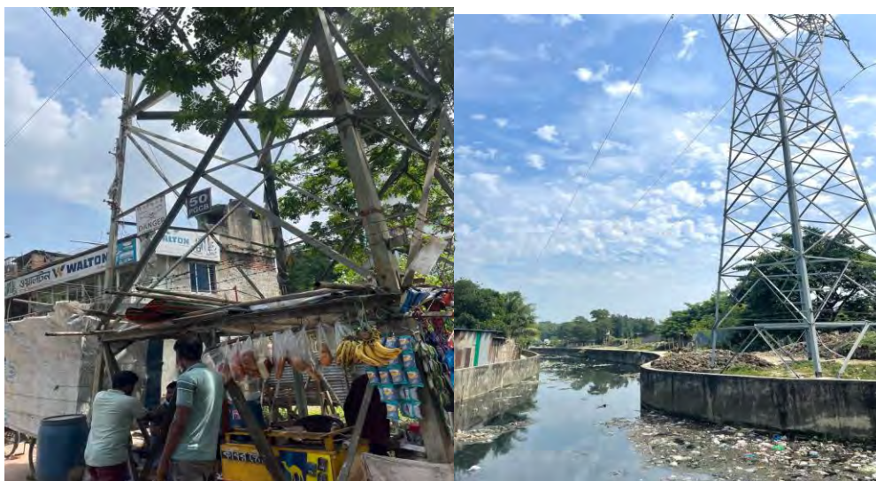
Figure 4: High Voltage Transmission Line
