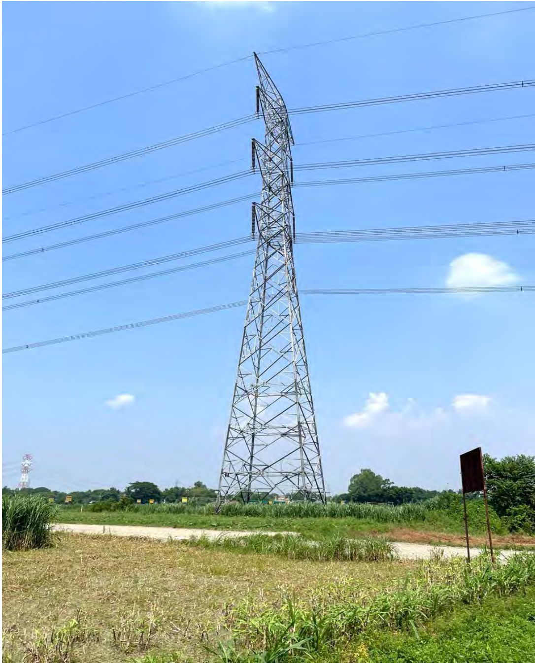
Figure 5: Greenfield High Voltage Transmission Line
