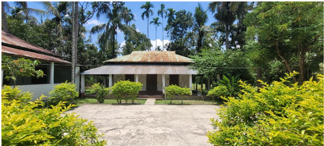
Figure 14: Tajuddin Ahmad's house located adjacent to the site (Source: author)
