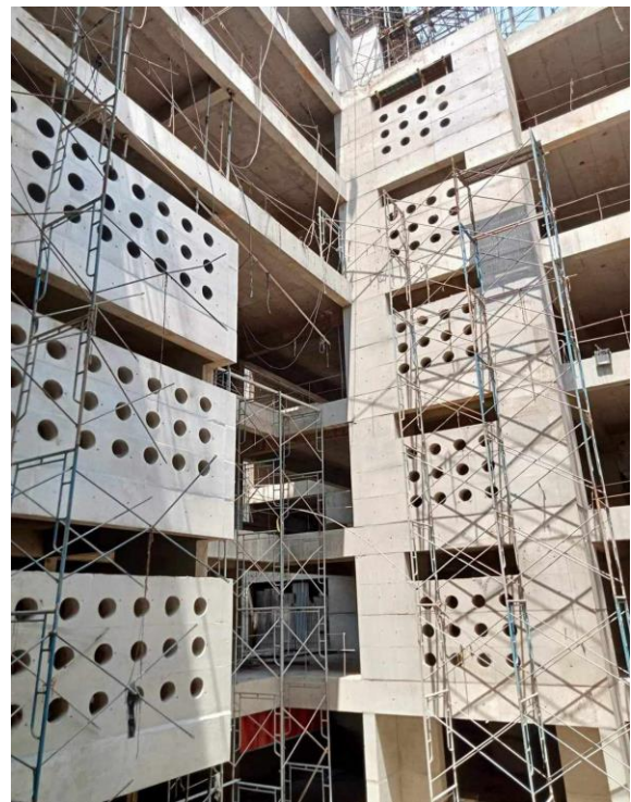
Figure 10- Project under construction, Source: AUST project's site office.
