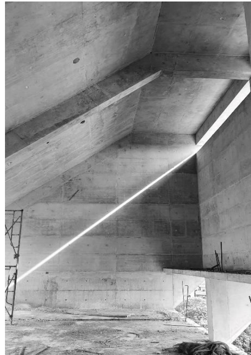
Figure 7- Project's inside view, Source: AUST Project's site office.
