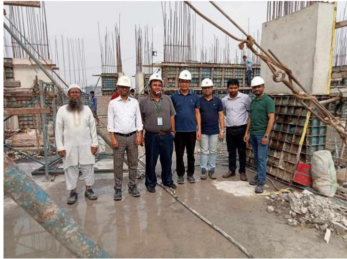
Figure 8- Site visit with authorities, Source: AUST project's site office.
