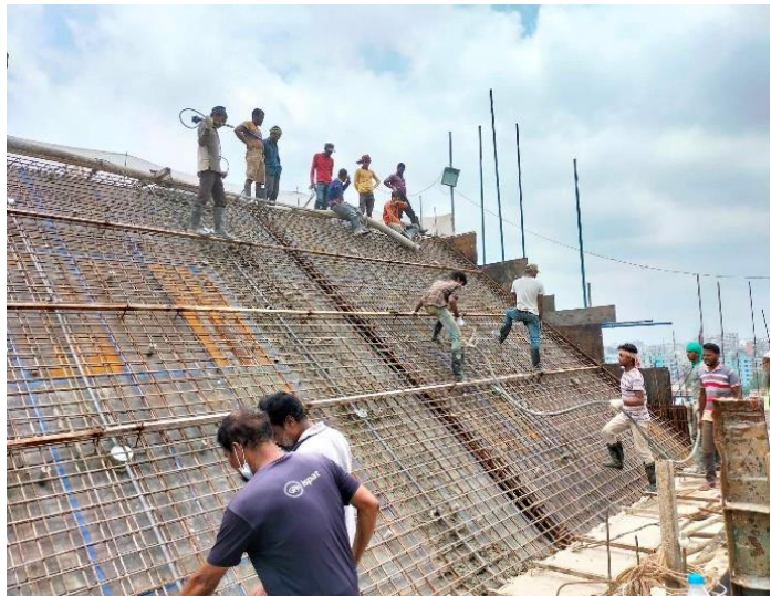
Figure 9- Monitoring during slab casting, Source: AUST site office.
