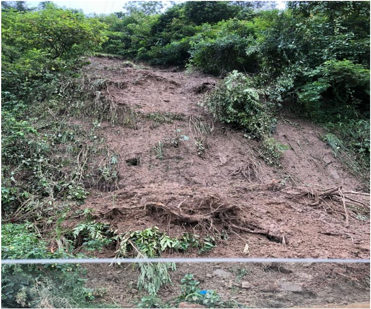
Figure 10 Debris flow after continuous rainfall, (Author, 2022)
