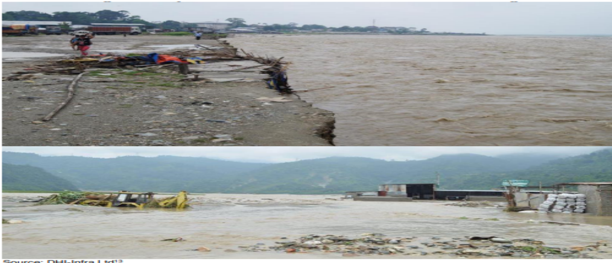
Figure12 July 2015 flood inundation and interal erosion damage
