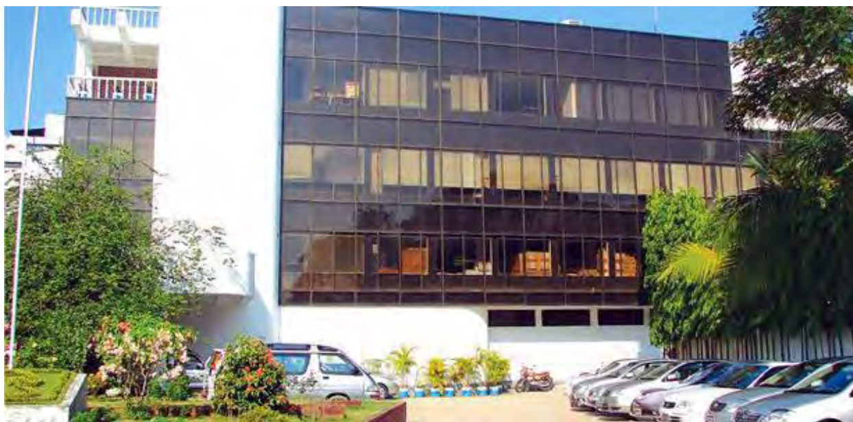
Figure 05: Part of Pabna Unit of SPL.
