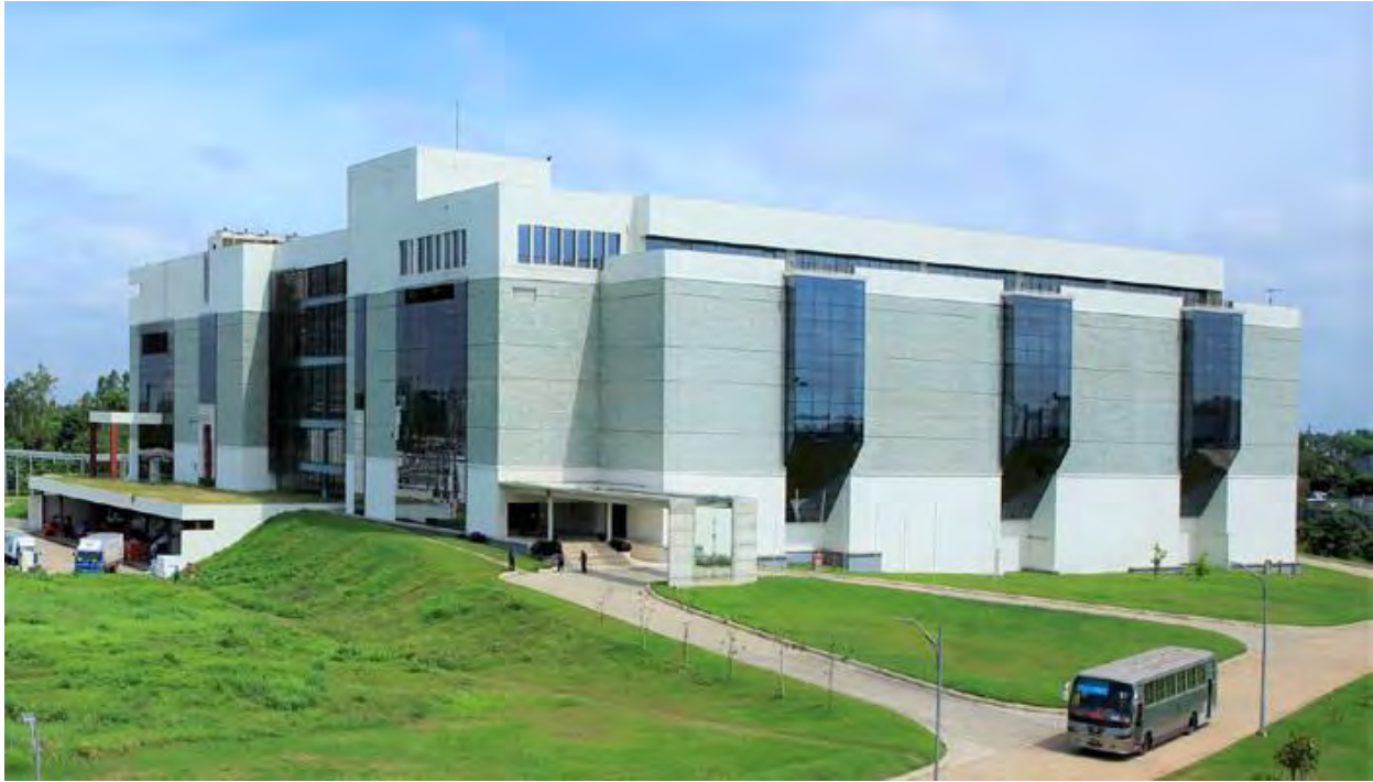
Figure 04: Part of Dhaka Unit of SPL.
