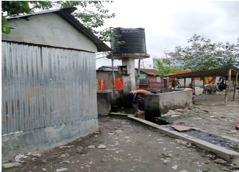
Figure 3: Bathhouse near drainage system
