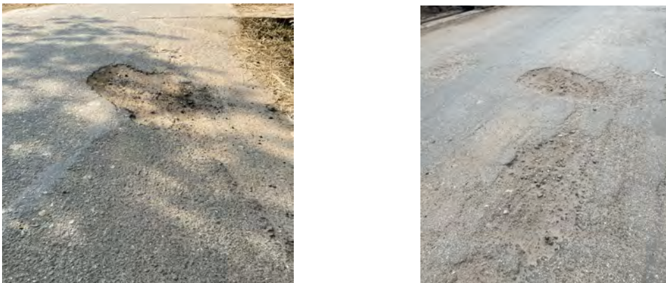
Figure 1.1: Pothole samples from our dataset
