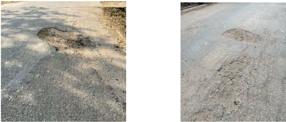
Figure 4.2: Pothole samples from our dataset
