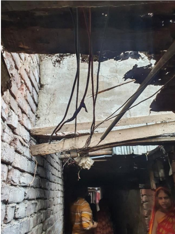
Fig 32: Exposed illegal electrical wires with poor connections and hose pipes used to supply gas within the slum community (Site survey, 2021)
