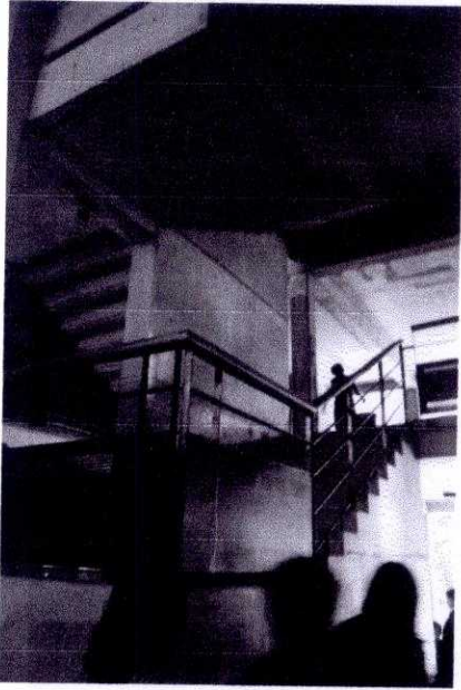
Fig 16: stair (source author)
