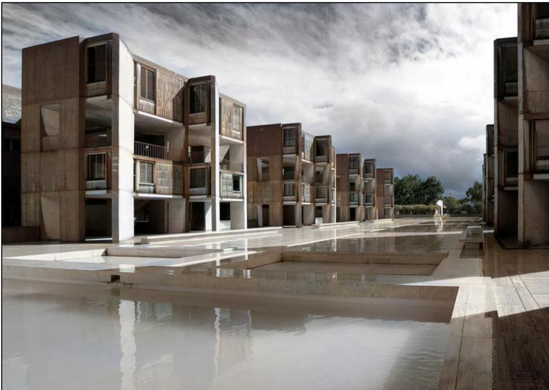
Figure 55: The view east, revealing the buildings' teak elements, saw tooth design and reflecting pool
