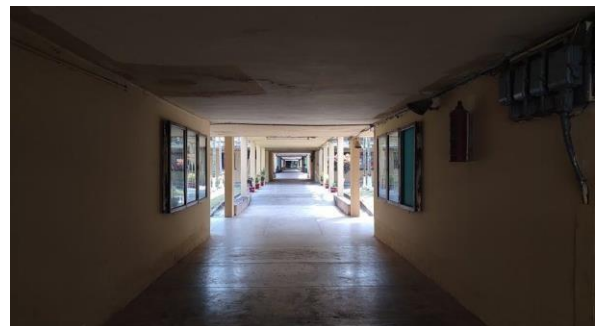
Figure 33: Corridor of main Building
