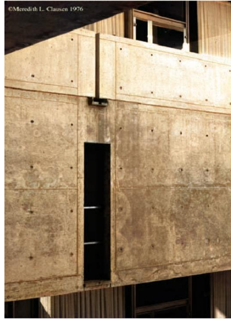
Figure 62: Concrete Walls Used
