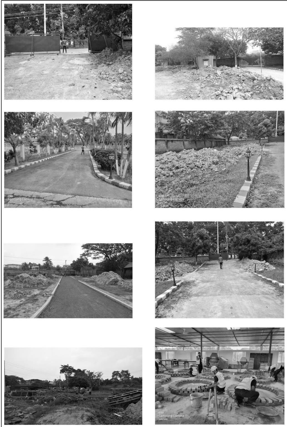
Figure 31: Images of Existing Site Condition
