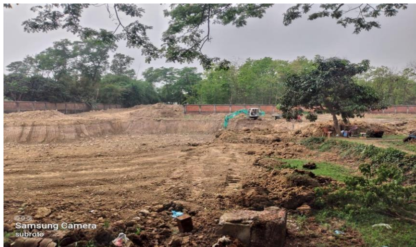
Figure 19: Ongoing Pond excavation
