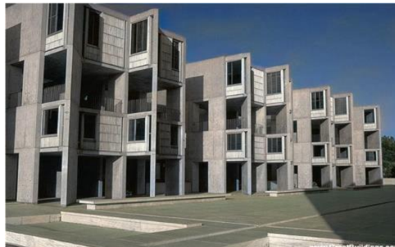
Figure 67: External Photo with Facade
