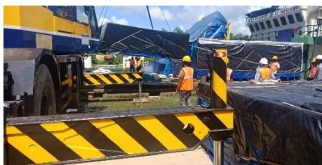
Figure-9 Downloading the Heavy Materials from Berge
