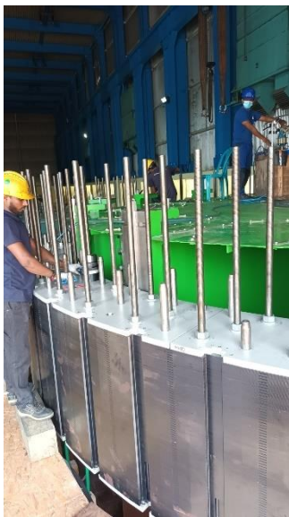
Figure - 6 Rim Sheet installation with Rotor Spider
