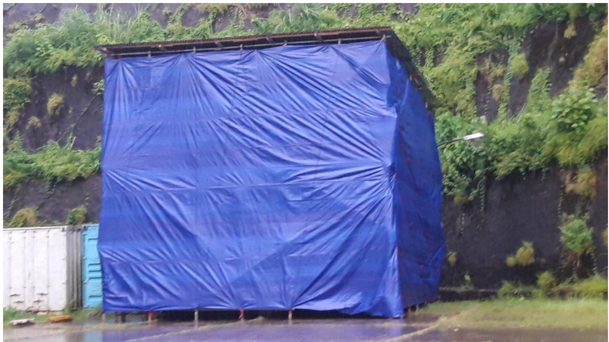
Figure -11 Storage of heavy materials
