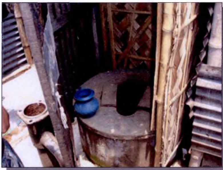
Pic-27 A pit type toilet used in Korail Beltola slum
