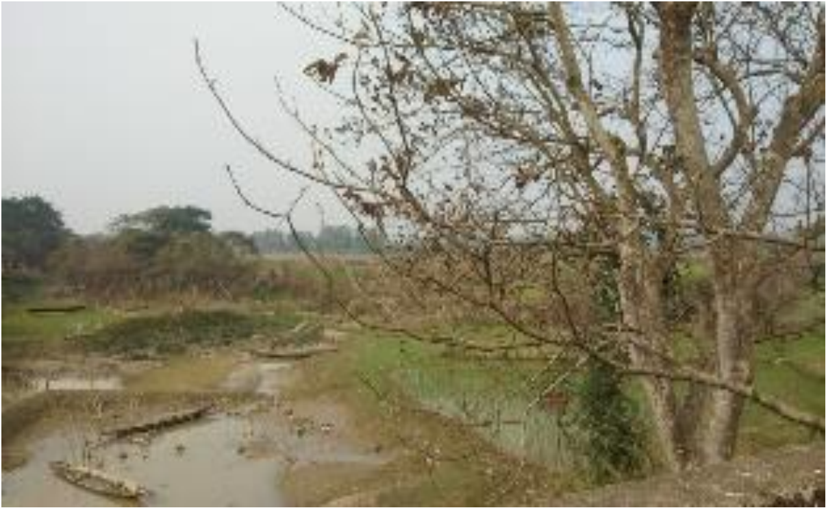
Fig 3.8.3: View of the canal in dry season (winter)
