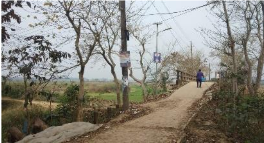
Fig 3.8.1: View of road (Donokandi road) and the culvert)
