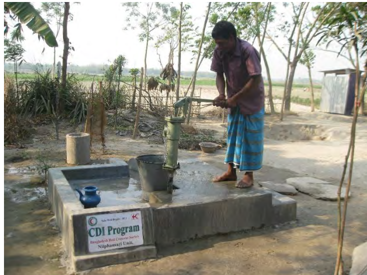
Figure 2: Tube-well with Elevated Platform
