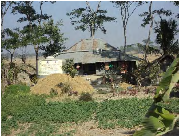
Figure 12: Existing RWHS in Sarabad
